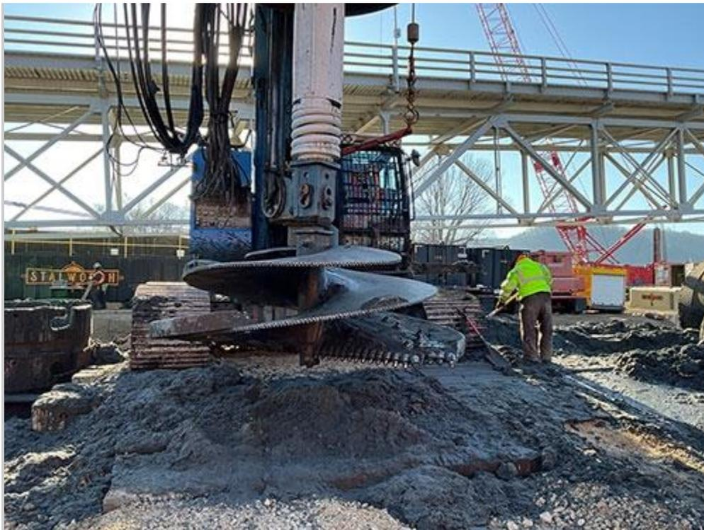
*Creating support for the new bridge ... The photo above shows the drill rig and auger used to dig the soil and sand out of a temporary casing by screwing the auger into the material and lifting it out of the hole near the existing Black Hawk Bridge. This process is used to create the shafts that will then be filled with concrete to create the supporting infrastructure of the new bridge at Lansing. Photo courtesy of the Iowa Department of Transportation.*
